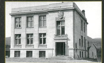
Courthouse - Corner Brook 1926
